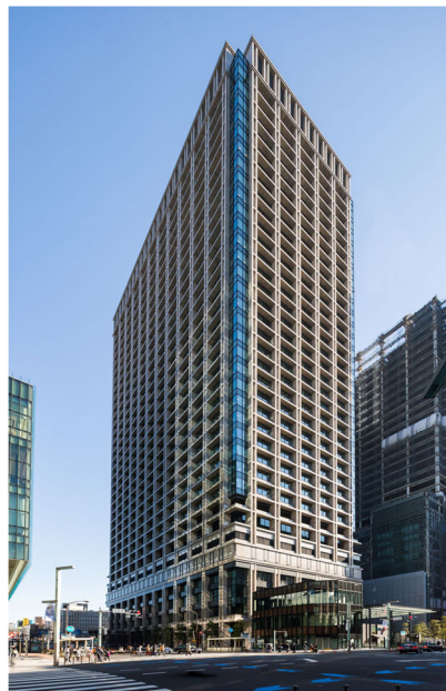
Tokyo Nihonbashi Tower
